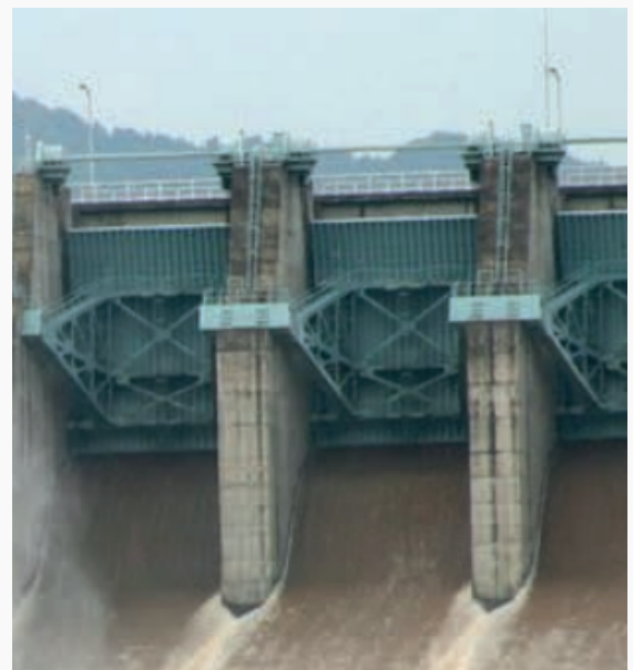
Daecheong Dam is located on the Geum River. It withholds a reservoir of 1,490 million cubic metres and has a generating capacity of 90 MW.
