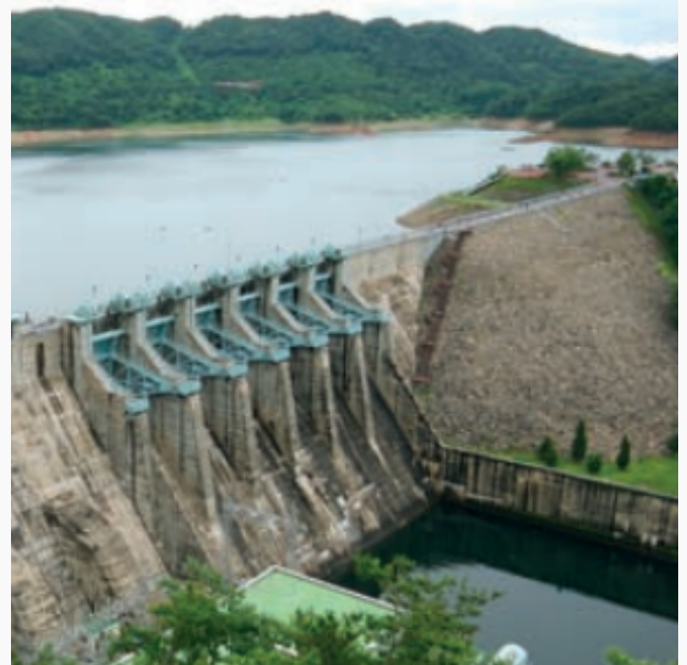
Imha Dam is located on the Banbyeoncheon River. With a capacity of 595 million cubic metres, it supplies water for 7.5 million people and industrial users.
