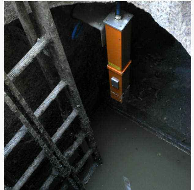
ROW installed and monitoring for oil spills on a stormwater channel
