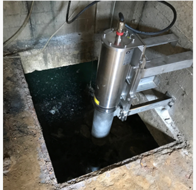
ROW installed and monitoring for oil spills on a stormwater main
